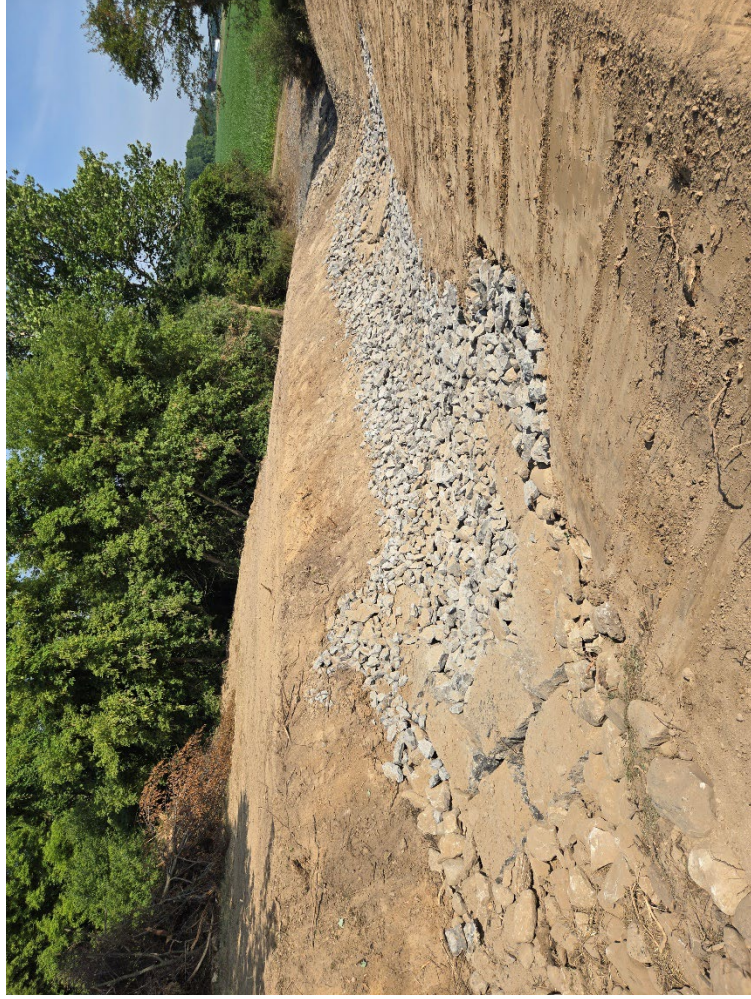
Photo 2: During construction with side slopes shaped and rock installed.
