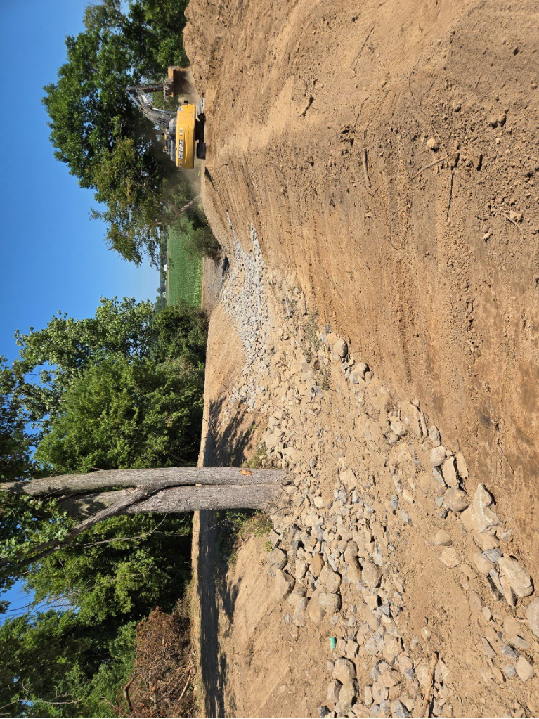
Photo 2: During construction with side slopes shaped and rock installed.
